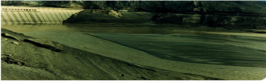
Fig. 1- Accumulated sediments behind the wall of Sefidrood dam
